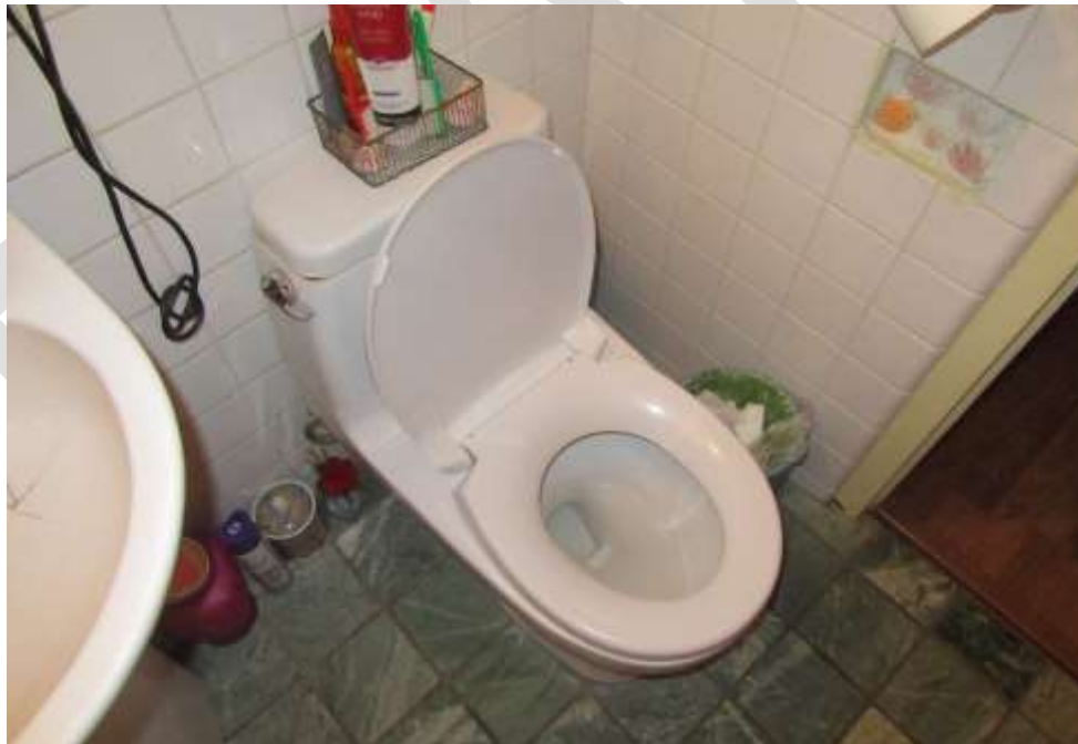
Typical Apartment Toilet
