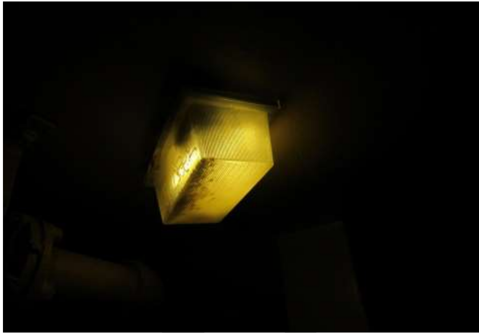
Typical Stairwell Lighting Fixture
