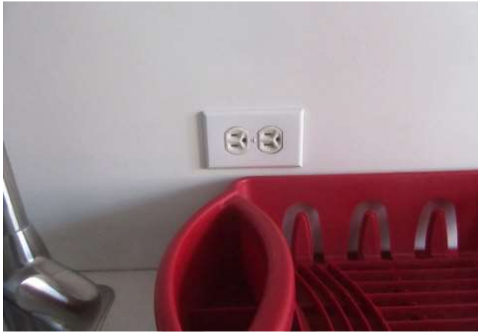
Apartment Non-GFIC Outlet in Kitchen
