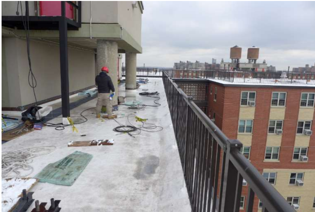
Building 2- Roof and Bulkhead
