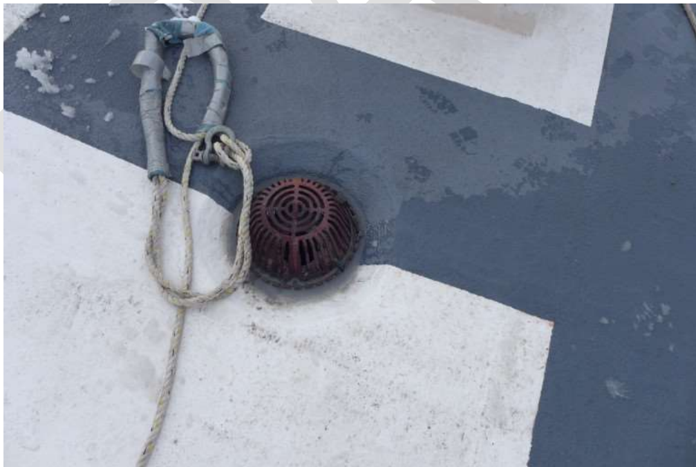
Building 2 – Roof Drain
