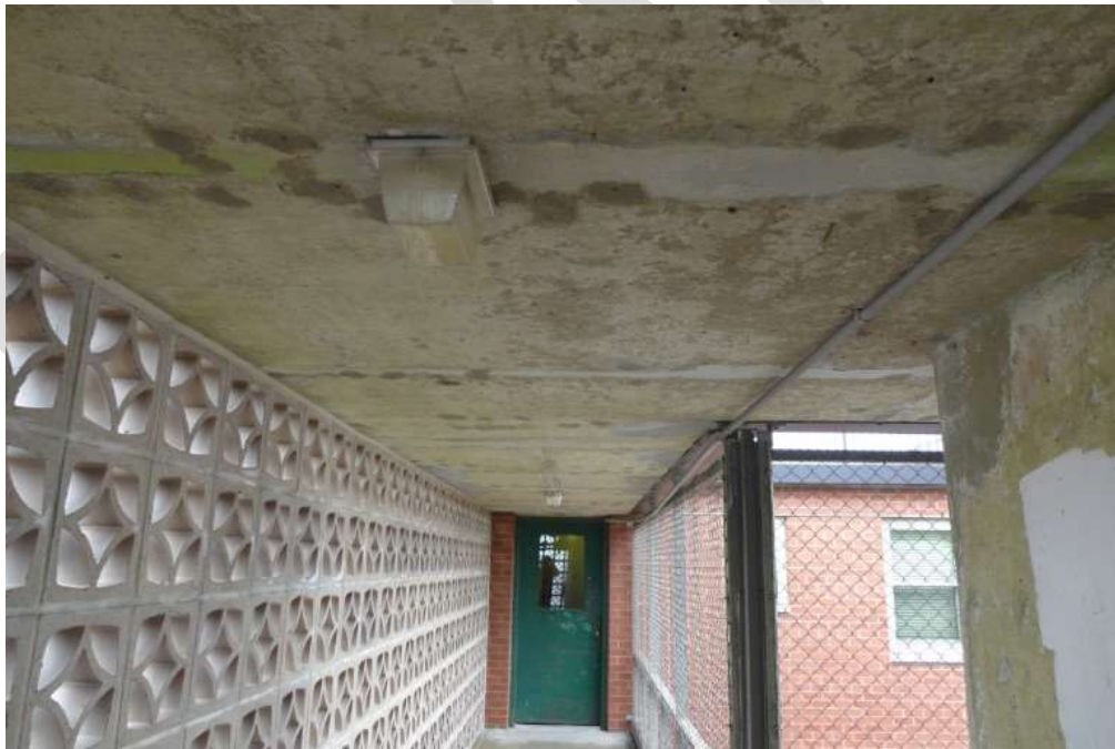
Typical exterior walkway and entrance door to apartment wings.
