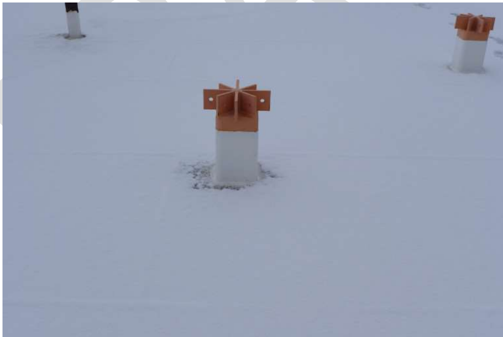
Scaffold tie-back installed during roof project.
