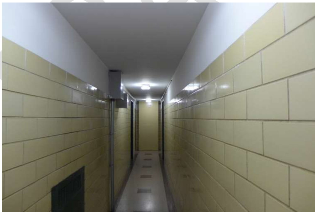
Typical interior hallway at apartment wing.
