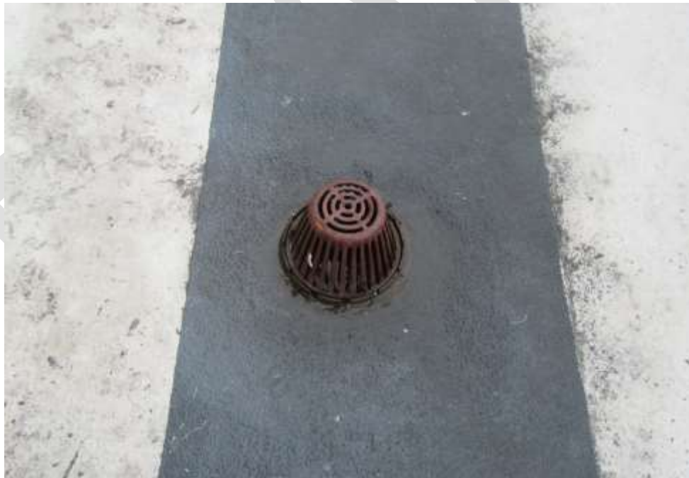
Typical Roof Floor Drain
