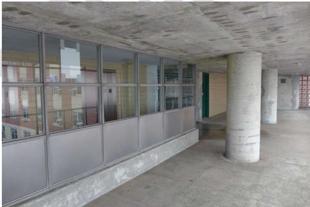
Typical elevator lobby at cores.
